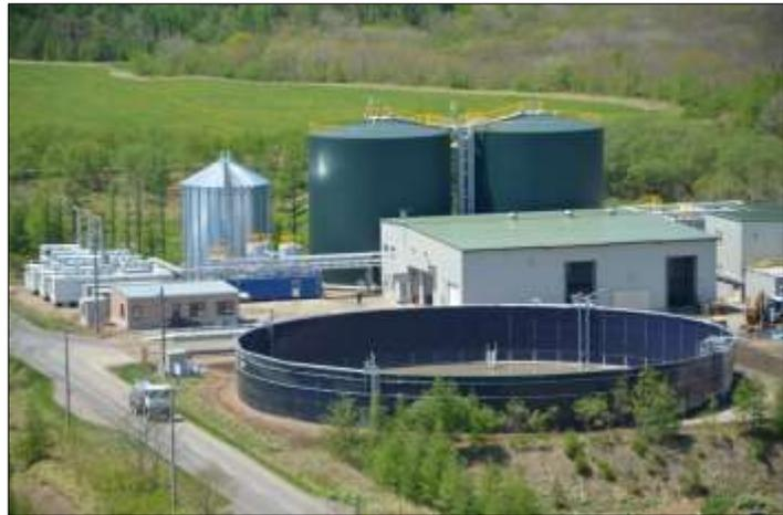
at the plant with high herbage content. The odor problem was resolved, methane production increased from 40% to the industrial norm of 60%, and power production rose from 100 kW/generator to reach full 300 kW/generator capacity.
