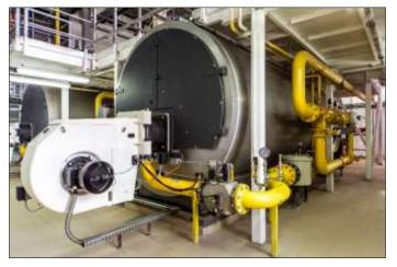
providers can perform dry layup of boilers, the Boiler  $Dragon^{TM}$  uses Vapor phase Corrosion Inhibitors  $(VCI/VpCI^{\mathbb{R}})$  to protect the internals of boilers and steam components from corrosion during short or long-term preservation periods. Unlike the Boiler Lizard<sup>®</sup>, Boiler Dragon<sup>TM</sup> will now be the go-to option for easy and effective dry layup of the largest boilers and their steam components surpassing 10,000 gallons (38,000 L) in volume.
