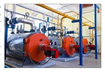
Cortec's Boiler Lizard® provides a simple, reliable, and effective way to properly preserve both boilers and deaerators for short and long periods of dry layup. Boiler Lizard® eliminates the need for other forms of protection such as silica gel, nitrogen blankets, and hydrazine, which can be labor intensive and, in the case of the last two, even dangerous.
