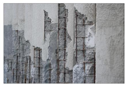
importance of service life prediction models and Migrating Corrosion Inhibitors (MCI®) in helping engineers achieve a structure's desired lifespan.
