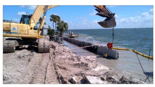
(based on mix components and the marine environment). This fell far short of the property owner's wishes. Adding MCI®-2005 into the mix design tripled the predicted service life of the original mix to 46.9 years until the first needed repair.
