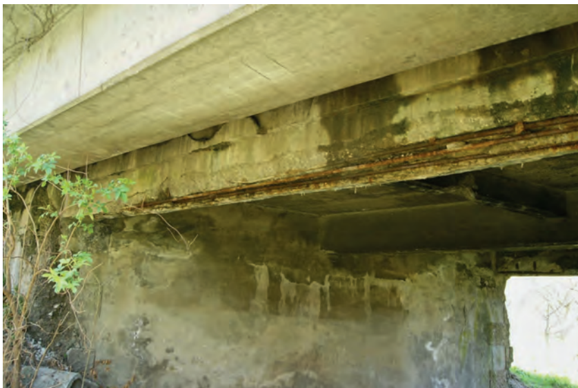
Below: Edge longitudinal girder – level of damage (left) and after (right).
