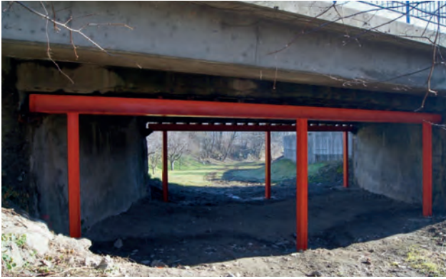
Above: Temporary support of the Lomost Bridge edge girders from October 2021 until full bridge repair works started.
