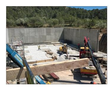
A water consortium that had previously had many corrosion problems wanted an innovative solution for a new reservoir they were building. MCI®-2005 concrete admixture was dosed at 0.6 L/m³ in a total of 1500 m³ of concrete forming the rectangular reservoir. This was an ideal solution because of their need for better durability from the start, as well as a product that could be used in a structure holding drinking water.
