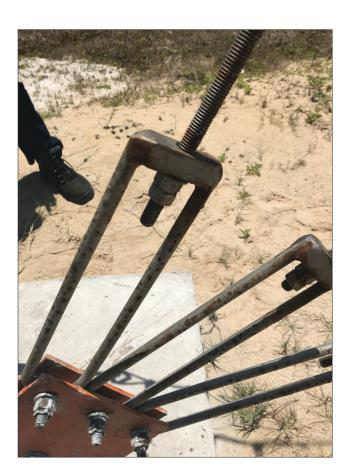
A corrosive environment of strong wind and blowing sand near the ocean led to corrosion on guy-wire clamps anchoring a cell tower in Brazil. The solution was to brush off loose rust, clean the clamps with VpCI®-418, and coat them with VpCI®-368, a wax-like, removable coating. This will be an important step to mitigate future corrosion in such a severe environment and thus prolong the service life of the critical components that keep the cell tower standing safely.
