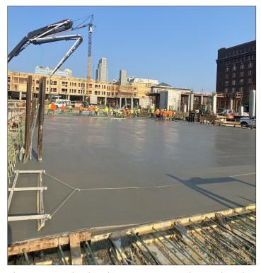
The Mercantile development in Omaha, Nebraska, included a four-story post-tension (PT) parking garage with a 100-year service life design. The use of deicing salts in the region is heavy during the winter, and freeze-thaw action allows chlorides to penetrate the concrete more quickly, so a corrosion inhibitor was needed. After a recent bad experience placing a concrete mix with calcium nitrite corrosion
