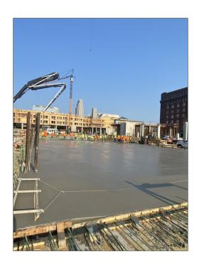
In 2021, a new mixed-use complex in Nebraska called for the construction of a four-level post-tension (PT) parking garage with a 100-year design life (before the first corrosion-related repair). Adding a corrosion inhibitor was essential because of the high corrosion risk from frequent winter freeze-thaw cycles, excessive ice, and heavy deicing salts.
