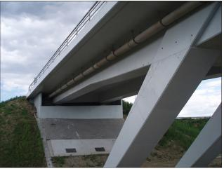
A Croatian overpass needed corrosion protection and a better appearance. The concrete surface was therefore cleaned and dried before workers applied a solution of MCI®-2020 Powder by brush and left it to dry for two days. The final step was to apply MCI® Architectural Coating (tinted grey) for additional protection and an improved appearance in the natural landscape.
