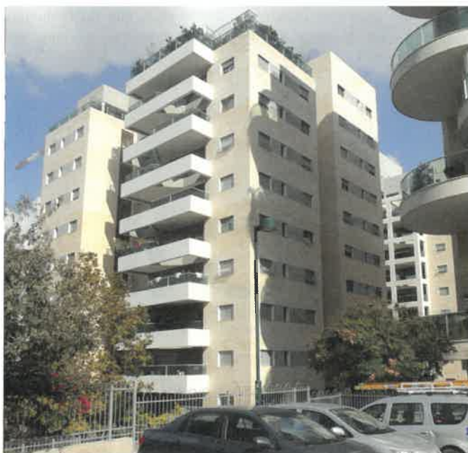
Fig. 2: Stav Street residential building after repairs completed (image courtesy of Glimmer Industrial Consultation)
