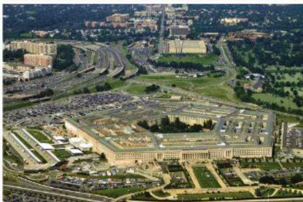
MCI® 2020 was chosen for renovation of Pentagon and has won International Concrete Repair Institute Award for the best repair project.
