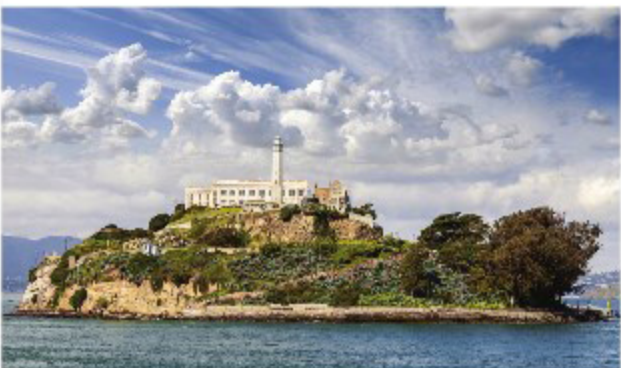
MCI 2020 was used for restoration of Alcatraz Island, the site of the Alcatraz Federal Penitentiary, located in the center of San Francisco Bay and surrounded by salt water and fog year-round. The National Park Service [NPS] selected MCI® 2020 to inhibit corrosion after loose, spalling concrete was removed.
