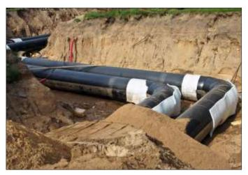
Interestingly, CorroLogic® VpCI® Filler gel is also electrically conductive, allowing it to be used in concert with cathodic protection (CP) to deliver the cathodic current to the carrier pipe. However, unlike cathodic protection, it does not require a constant source of electricity, and it continues to protect the pipeline even if the CP electricity source should fail.
