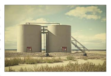
(Middle East & North Africa) region is not an exception. Ingress of chlorides and other corrosive species from the native soil and groundwater through the tank pad, along with the presence of bacteria such as SRB, are believed to be the main causes for soil-side corrosion. Airborne chlorides and moisture can seep into the under-tank environment through the chime area, causing annular plates to corrode.
