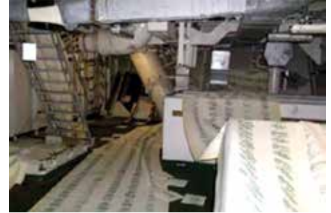
After entering a two year layup period, the internal volumes of the rooms of HMS Albion ship were protected using Cortec's VpCI®-132 and VpC®-137 foam.
