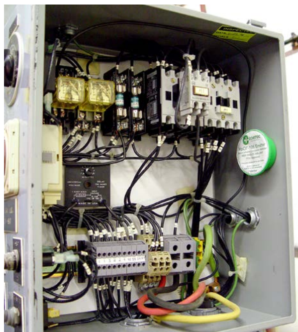
Illustration of how Vapour phase Corrosion Inhibitor technology forms a protective molecular layer on metals in an enclosed space. Image courtesy: Cortec Corporation.
