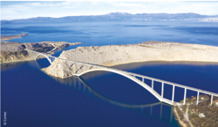
Figure 1: Krk Bridge is reinforced concrete arch bridge connecting the Croatian island of Krk to the mainland and carrying over a million vehicles per year.
