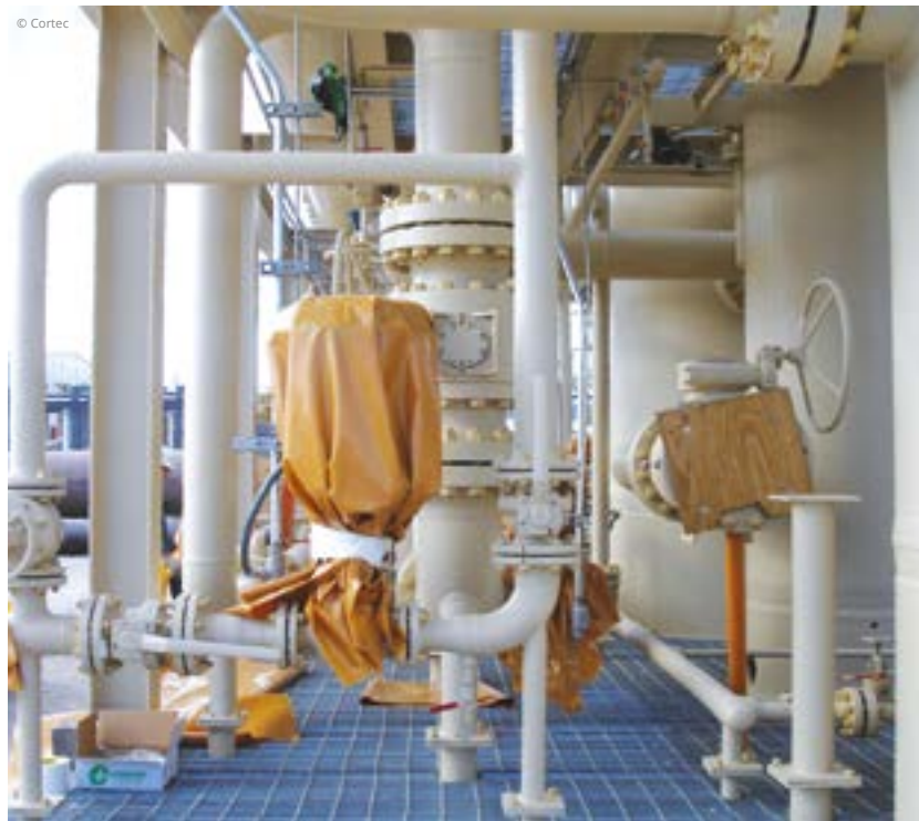
Figures 1 and 2 - Equipment, pipes, flanges, and units wrapped in MilCorr VpCI Shrink Film.
