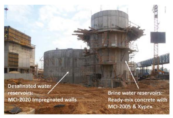
MCI®-2020 was used to protect desalinated water reservoirs and columns at a desalination plant after insufficient concrete coverage of rebar was discovered.
