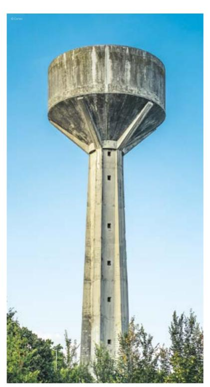
Reinforced concrete potable water structures are at higher risk for corrosion because of constant exposure to moisture.
