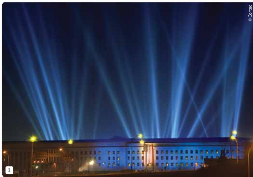
1 MCI®-2020 was chosen for renovation of Pentagon and has won International Concrete Repair Institute Award for the best repair project.
