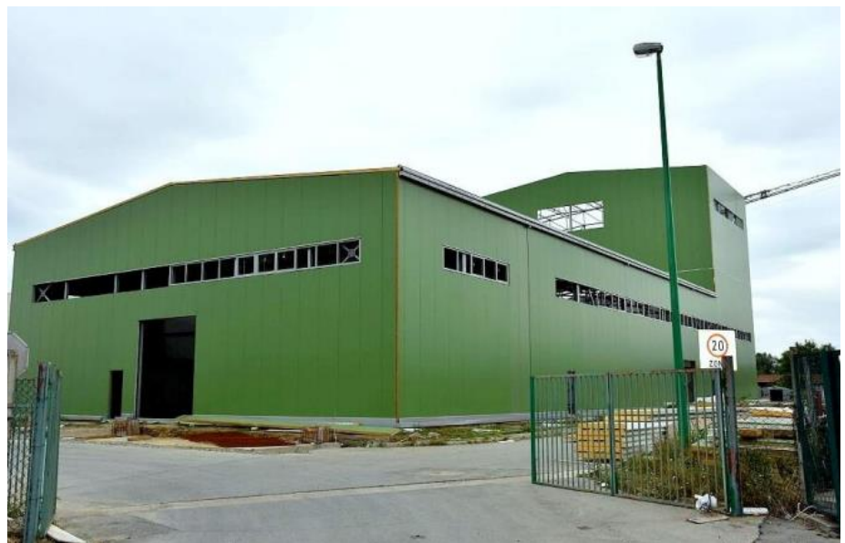
Result of growing business: New EcoCortec plant facility is set to open in October 2018 during Cortec European Sales Meeting.
