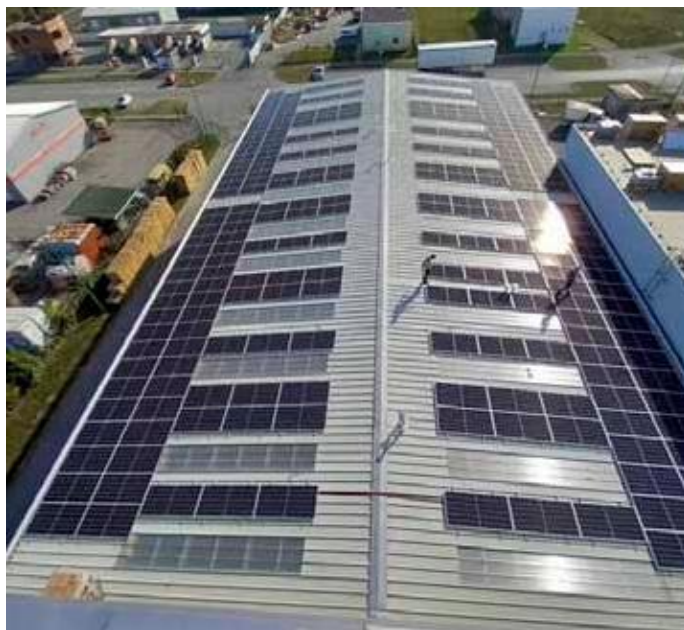
Installing solar panels on the roof of EcoCortec® plant.
