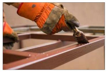
performing water-based DTM (direct to metal) permanent coatings is EcoShield<sup>®</sup> 386, which has been able to provide outstanding corrosion protection in salt spray chamber testing. Cortec<sup>®</sup> has recently expanded this unique portfolio of water-based anti-corrosion coatings by developing a new fast-dry version called EcoShield<sup>®</sup> 386 FD.
