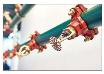
At least two methods of Vapor phase Corrosion Inhibitor application exist. One option is to use VpCI® fogging fluid to deliver the corrosion inhibitors immediately through the dry pipes. The other employs more gradual vapor dispersion by placing dry Vapor phase Corrosion Inhibitors in a housing connected to a pressurized air system that constantly circulates the protective vapors through the piping. This comprehensive
