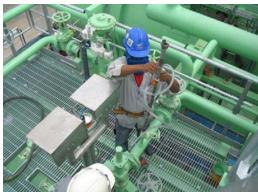
Veto Aible in Banchang, Thailand, needed corrosion protection for the internal surfaces of piping supplied to the Cinguetti Project. The company found out that  $VpCI^{@}609$  was the most cost effective solution to the internal corrosion problem. It was easily applied and provided 24 months of continuous liquid, vapor phase and interface protection.
