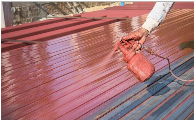
On the other side of the coin, the customer's application process can be a huge gamechanger—not because of something wrong with the coating but because different application methods affect the same coating differently. For example, the use of an airless sprayer versus the dip coating process means viscosity may need to be adjusted to make the coating flow more smoothly through the
