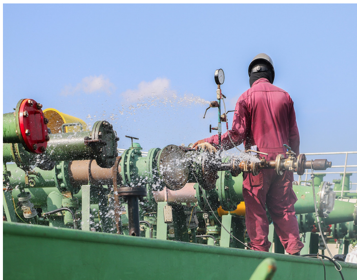
Figure 1. The very process intended to confirm vessel integrity can undermine it by introducing moisture and leaving metal surfaces vulnerable to corrosion. (Image courtesy of Cortec Corp.)
