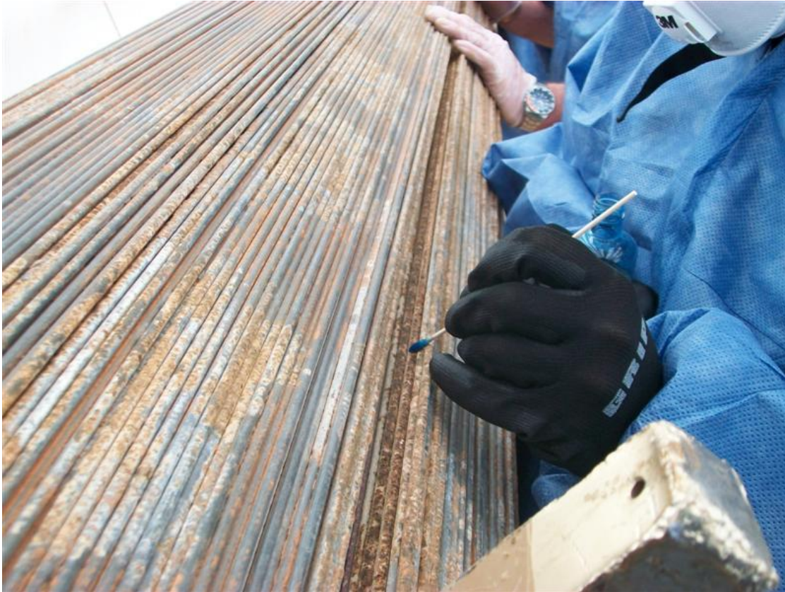
Figure 3: Swab test for inhibitor during cable inspection.
