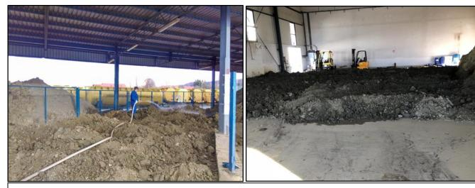
BCP35S and BIOSURF were mixed with fresh water and sprayed on the surface of the contaminated soil, which is simultaneously agitated.
