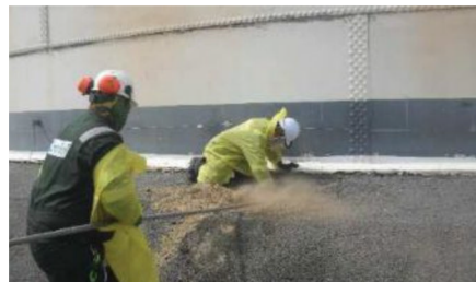
Air lancing to remove sand. Image courtesy of CorrTrol.
