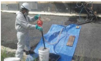
Injecting VCI. Image courtesy of CorrTrol.
