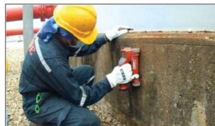
Before drilling through the concrete to create openings for VCI injection and ER probes, workers scanned the concrete ring wall to locate and avoid embedded reinforcing metal. Image courtesy of CorrTrol.
