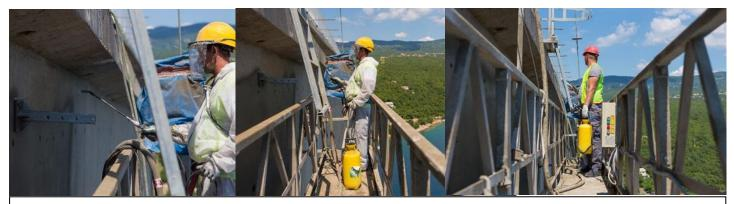
Application of MCI® -2020 will stop further corrosion of reinforcing metals and extend the service life of the bridge.
