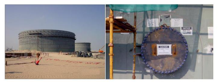
Cortec® proposed this chemical system as an economical and environmentally responsible method of effective corrosion protection for interiors of carbon steel tanks subjected to hydrostatic testing using
