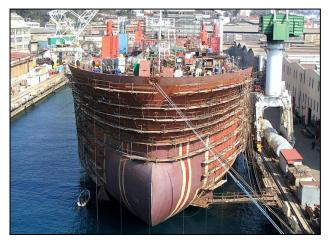
Optimal and smart corrosion protection is one of the key factors in the quality and price of the ship. Structures in shipbuilding, offshore and marine industries contain parts that are difficult to access or can even be completely inaccessible for quality and long-lasting protection. Parts of the ship structure are derived from a number of brackets, frames, stiffeners and reinforcements which makes them difficult for proper preparation and coatings protection.
