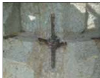
Left picture: Damaged steel bands. Right picture: CorrVerter® applied to the right side of the band; the coating has converted the corrosion into a protective layer.
