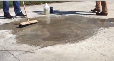
The video shows workers brushing MCI®-2061 concentrate onto the stains. then applying water to activate the microorganisms in the product. After leaving MCI®-2061 to biodegrade the hydrocarbons in the concrete overnight, they came back the next day and rinsed the concrete slab with water and left it to dry. The client was very satisfied with the cleaning results and ease of application – no blast cleaning required!
