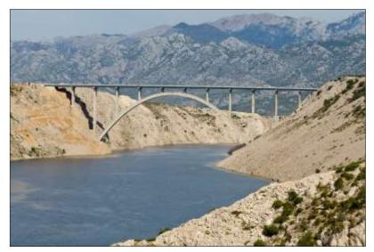
The Maslenica Bridge experienced concrete spalling and corrosion of reinforcing steel because of an aggressive environment near the Adriatic Sea. In addition to the use of MCI<sup>®</sup>-2020 on the entire concrete structure, CorrVerter® MCI<sup>®</sup> Rust Primer was applied to exposed rebar by brush after removing dirt, corrosion, and spalled concrete using a high-pressure water blast.
