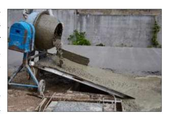
suppliers—who can simply calculate the right number of MCI® Grenades to toss into the concrete batch at the jobsite to get corrosion protection and extend service life.
