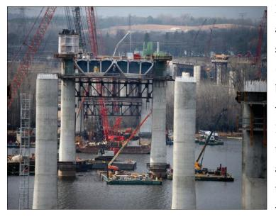
Because of its unique environment, the approximately one mile long crossing was specially designed as an extra dosed bridge (combination box girder and cable stay bridge) to minimize the environmental and visual impact of the structure on the St. Croix River Valley. As one of only two of its kind in the United States, it is a model of engineering and design ingenuity. Cable stays support the bridge at five pier locations in the river, while approximately 1,000 pre-cast boxlike
