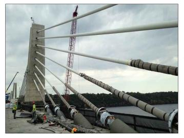
MCI®-309 can be easily fogged through posttension ducts using a low-pressure air hose after PT strands are placed in the duct. The powder vaporizes and adsorbs on metal surfaces, forming a protective molecular layer on the tendons. The layer helps reduce corrosion by inhibiting interaction with corrosive elements such as air, moisture, and chlorides. As a mixed inhibitor, MCI®-309 discourages both cathodic
