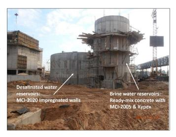
below the surface of the concrete within one month of application. It was <u>used to protect desalinated water</u> <u>reservoirs and columns</u> at a desalination plant after insufficient concrete coverage of rebar was discovered.
