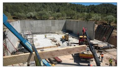
When constructing new potable water tanks out of reinforced concrete, engineers can specify MCI®-2005 or MCI®-2005 NS water-based corrosion inhibiting admixtures. These concrete admixtures meet all physical property and corrosion inhibiting requirements of ASTM C1582 and are very user-friendly for ready-mix suppliers. Unlike traditional calcium nitrite
