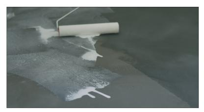
corrosives to enter and attack embedded rebar, starting a whole new cycle of expansion, cracking, and concrete deterioration. A silane sealer can help slow this process.
