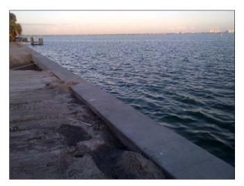
subtropical seaside environment, where the reinforced concrete would be constantly exposed to high-chloride seawater. However, the owner was confident that this high standard could be achieved by using MCI®-2005 to help extend the service life of the seawall.
