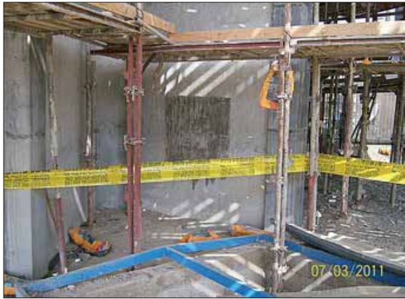
Demonstrating MCI®-2020 application on 1 Square Meter
