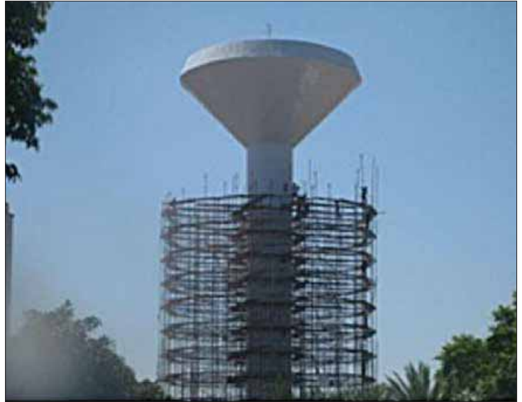
South Tower during application.
