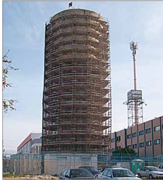
Holot Tower during restoration
