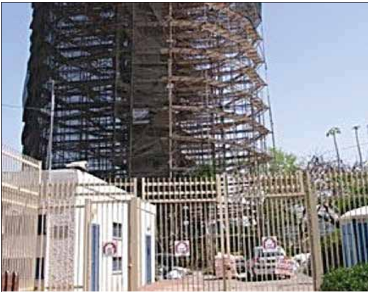
South Tower during application.
