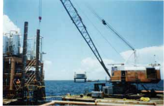
Piles being driven into the sea bed
