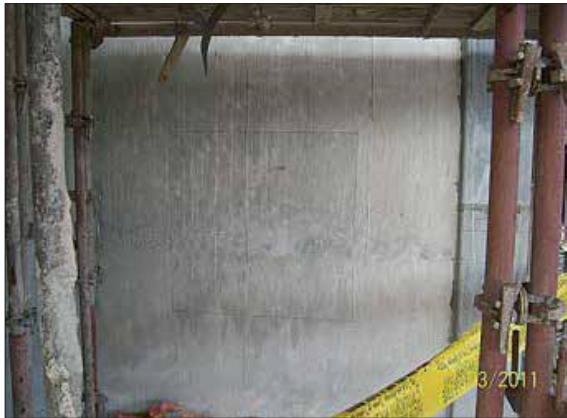
MCI®-2020 demonstration two weeks from application - almost undetectable
