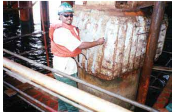
MCI®-2023 rebar coating applied on Pile-cap
