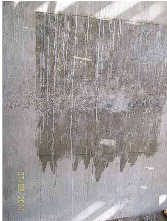
Demonstrating MCI®-2020 application on 1 square meter
