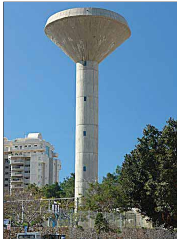
South Tower prior to application.
