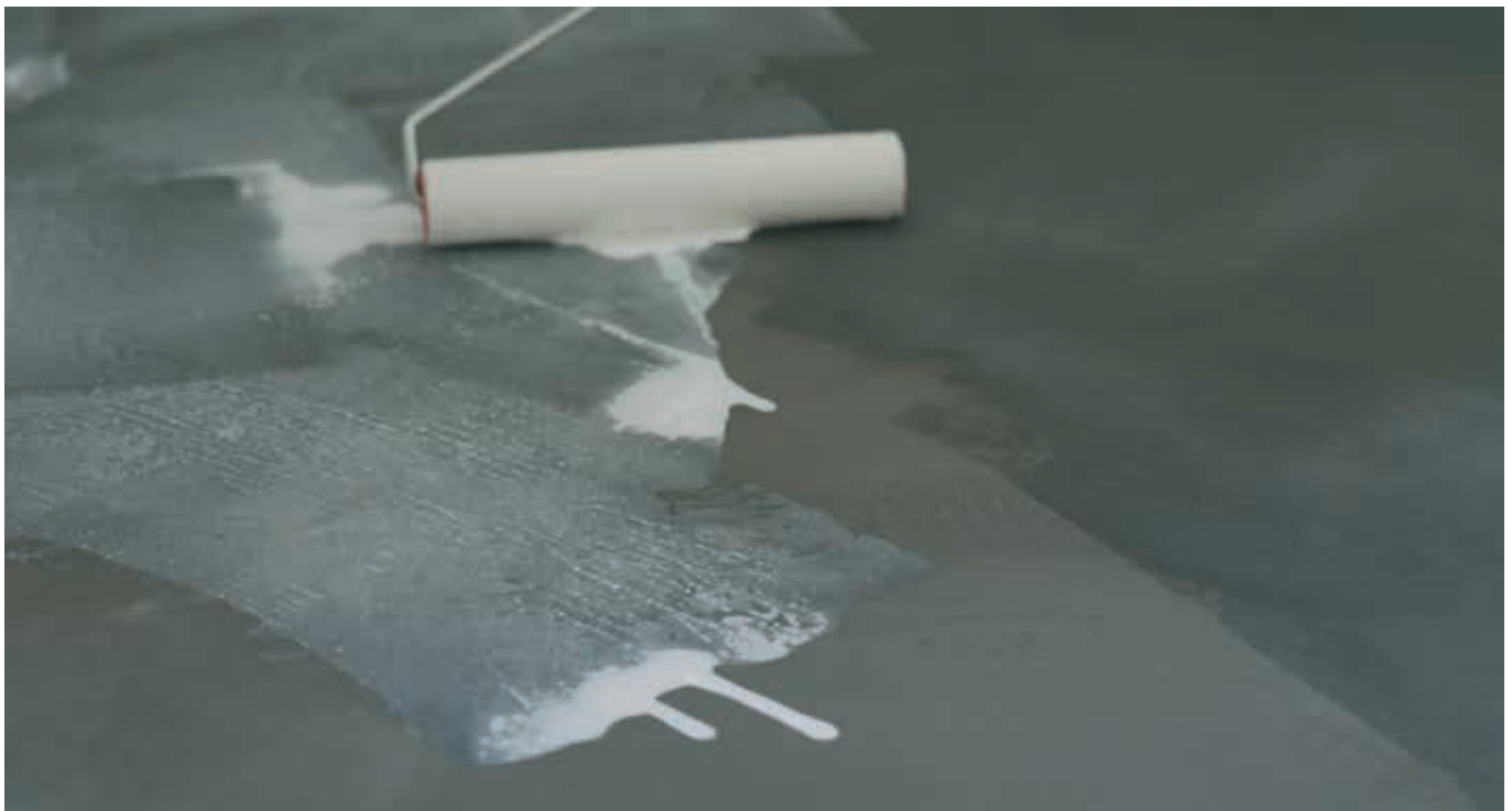
When applied, MCI® water repellents create a hydrophobic layer at the concrete surface to prevent intrusion of chlorides and carbonation, and to protect concrete from the ingress of wind-driven rain.
