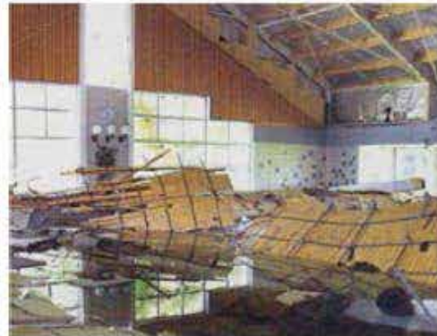
Figure 29: Collapse of suspended ceilings in swimming halls due to inappropriate stainless steel fastening elements. Failure by stress corrosion cracking. 41
