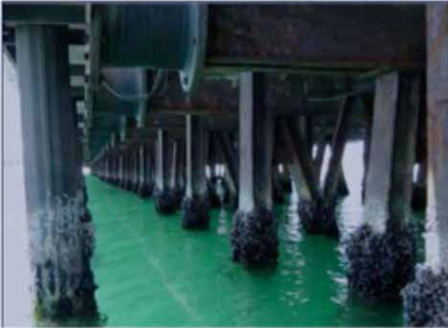
Figure 20: Marine corrosion of steel piles. 28
