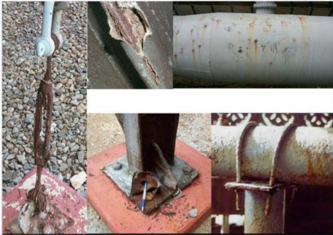
Figure 17: Corrosion of structural materials due to highly corrosive atmosphere in range of the plant. 26
