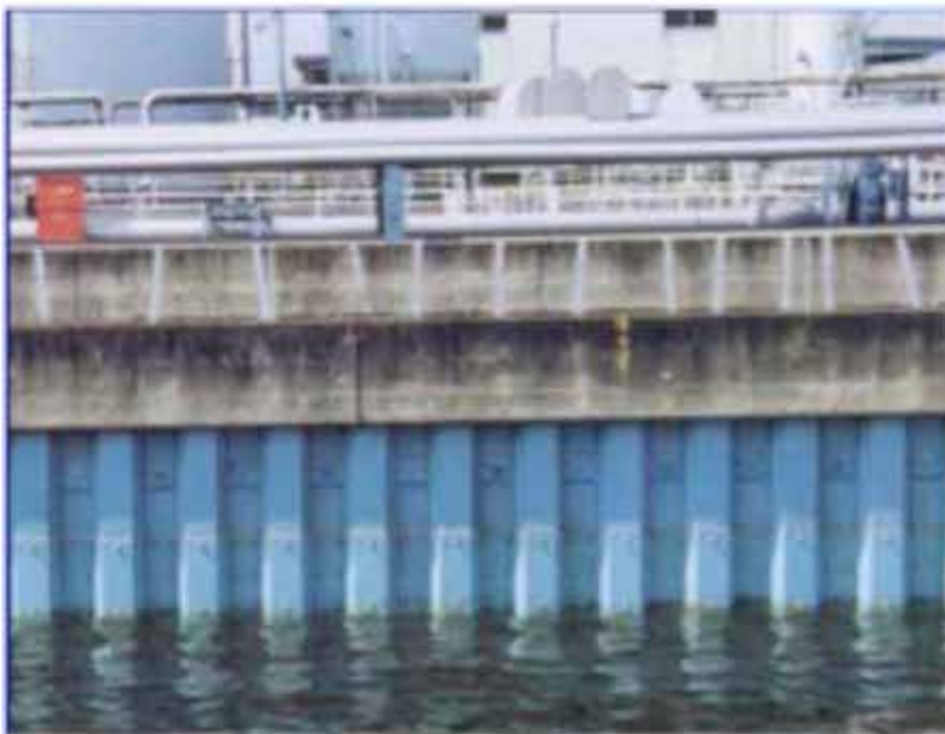
Figure 23: Underwater and splash zone coating. 29
