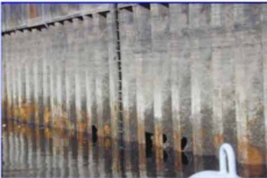
Figure 21: Low water zone corrosion of sheet pilings. 29
