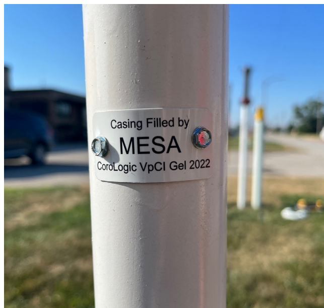
Figure 5. Sign on cased pipeline crossing vent indicates when the casing was protected by MESA. (Source: Cortec, courtesy of Eric Uutala)
