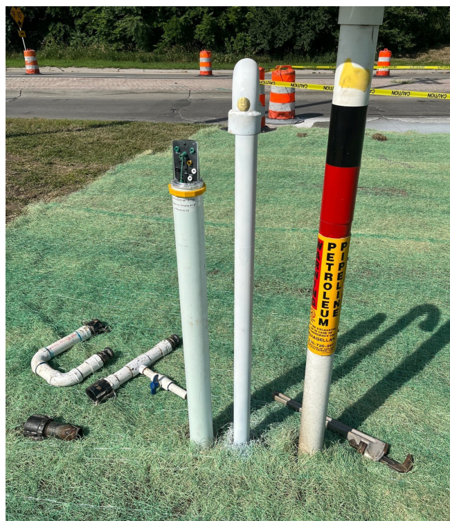
Figure 3. The centre pipe is the ventilation duct to the pipeline casing buried underground at this pipeline crossing. A similar vent on the 'low side' (ventilation to the bottom of the pipe) is where CorroLogic VpCI Gel application is ideal. The left pole is where the electrical potential can be measured to determine CP condition. (Source: Cortec, courtesy of Eric Uutala)
