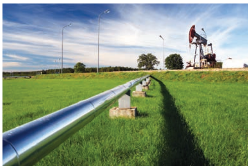
The solution will be deployed on pipelines in North Dakota
