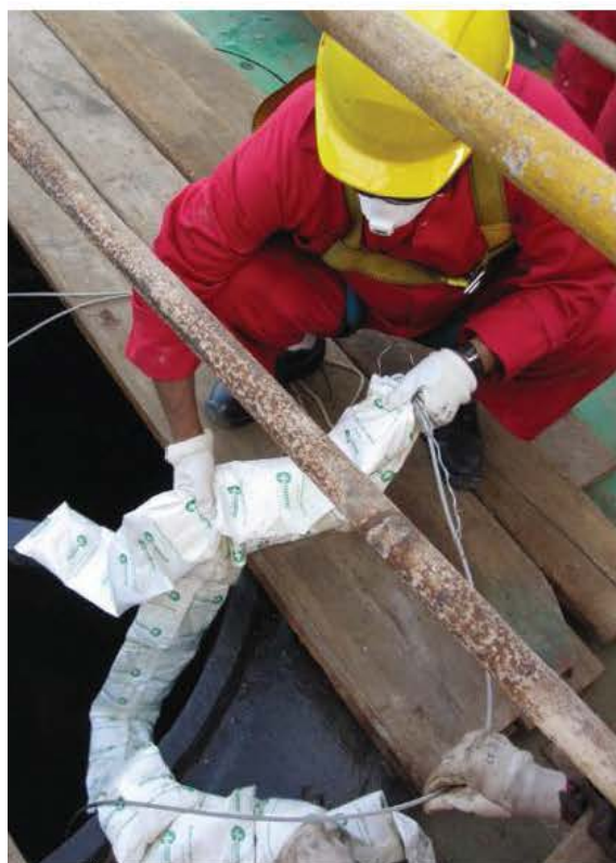
Figure 3: Corrosion inhibitor being applied to caisson legs.
