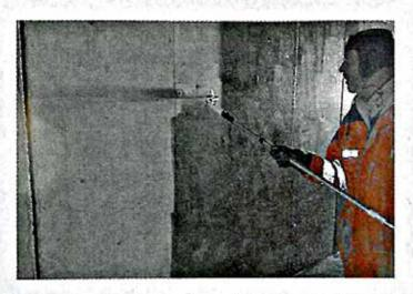
used over various types of masonry that are both coated and uncoated. It is a permanent coating that does not need to be recoated after graffiti removal. After 24 hours of first applying the coating, it can be tagged without affecting the graffiti resistance, and any graffiti can be immediately removed with a cold-water pressure cleaning. It can be reapplied at any time. 800/426-7832;
