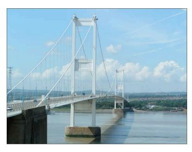
The Severn Bridge, in Wales, England, is a cable stay bridge maintained by the UK Highways Agency, and is an example of a bridge using this technology. The suspension cables on this bridge type are known to corrode over a long period of time. The first inspection of the main cables found they were corroded and had reduced structural strength. An acoustic monitoring
