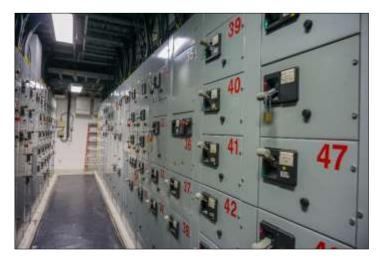
A number of basic equipment preservation strategies apply to almost any plant. For example, electronics and electricals should be protected from corrosion by placing the correct size and number of VpCI<sup>®</sup> Emitters into junction boxes and electronic cabinets depending on enclosure volume. A VpCI<sup>®</sup>-101 Device is good for small boxes of up to 1 cubic foot (28 L), and one VpCI<sup>®</sup>-111 Emitter protects up to 11 cubic feet
